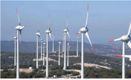
WIND POWER PLANT (WPP)
