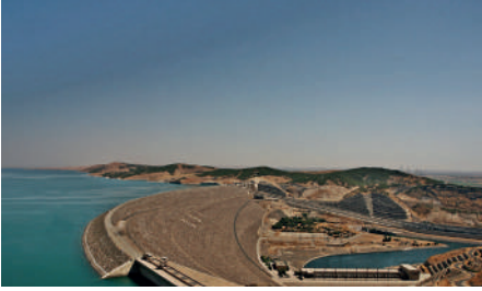
URFA SOLAR POWER PLANT (SPP)
