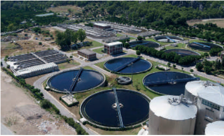
ANTALYA ASAT WATER TREATMENT PROJECT
