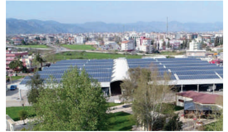
ANTALYA PAZARYERİ SOLAR POWER PLANT (SPP)
